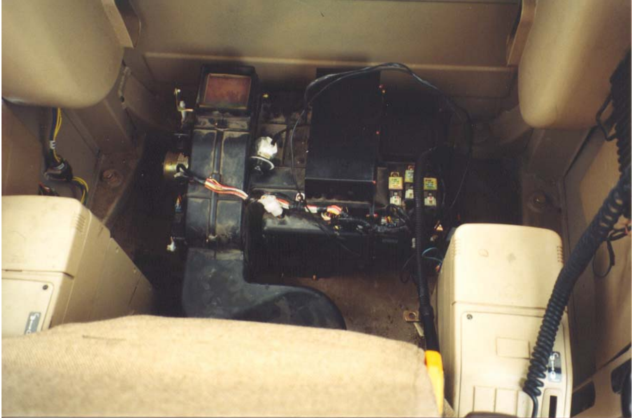
Evaporator/Heater assembly in place with thermostat inserted
